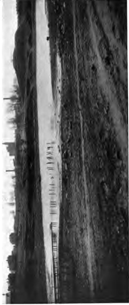
FIG. 7.—Topsoil Stripping, Piling, and Grading.
